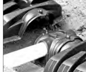
Optional: Fasten the end cap to the chamber with a screw at the top of the end cap.
