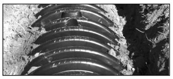
• Modestly compact the sidewall area backfill material by simply walking down the sides of the chambers. Sidewall compaction is important to begin the stabilization process of the soil, to support the chamber sidewalls, and help prevent fine sand migration into the chamber louvers. This procedure may be accomplished any time during the installation or covering process.
