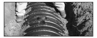
• All ARC chambers are H-10 load rated. Where vehicular loading is anticipated during installation of the system or construction of the facility, H-10 loading (16,000 lbs/axle) is achieved by backfilling with a minimum of 12" of properly compacted cover.
