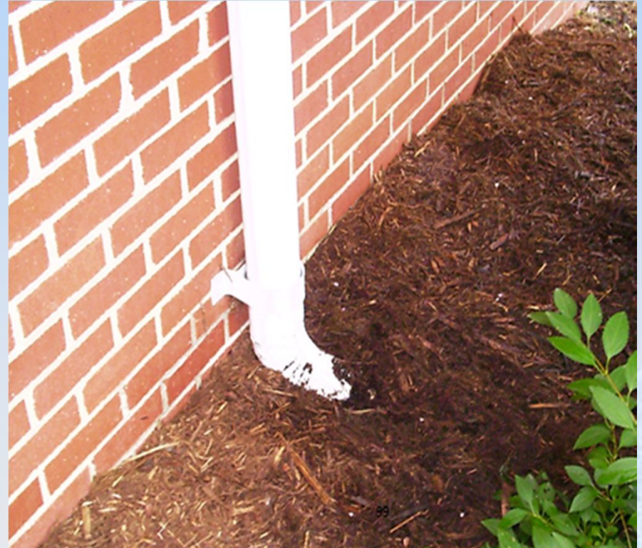
Ground water accumulation against the foundation
