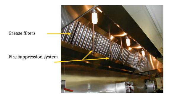
The National Fire Protection Association provides a resource for FOOD ESTABLISHMENTS to reduce the potential fire hazard of commercial cooking operations. Refer to the NFPA link below or your local/State Fire Protection regulations.
